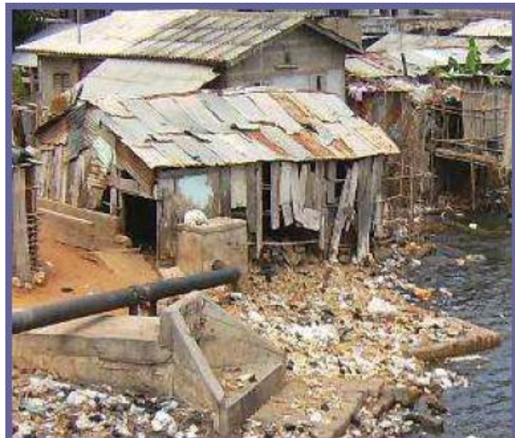
Diagram 2.1 : Outlet of rain waters or waste waters’ main sewer, drink water conduits stripped by erosion in an unhealthy environment on the banks of the Cotonou lagoon
