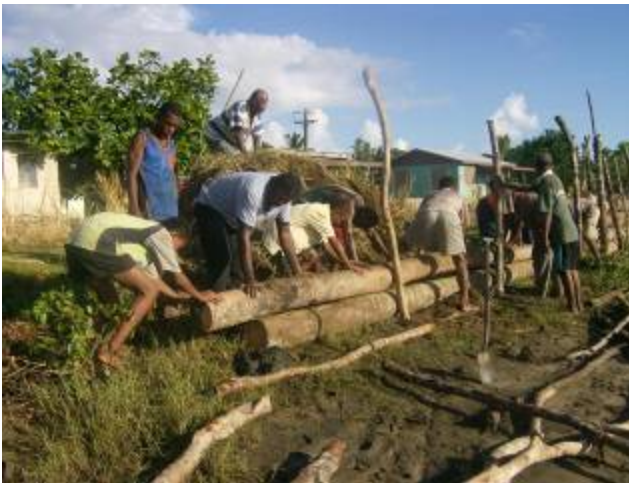
Construction of river bank protection structures using local materials, and planting of vetiver grass for bank stabilization (Buretu, Fiji – USP CBA project)
