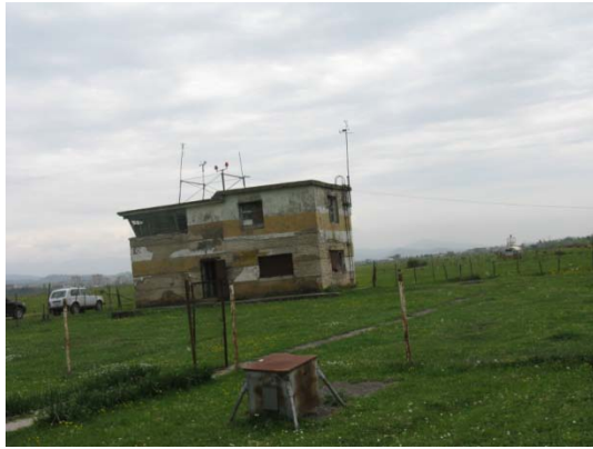
e) Hydrometric Station building station
