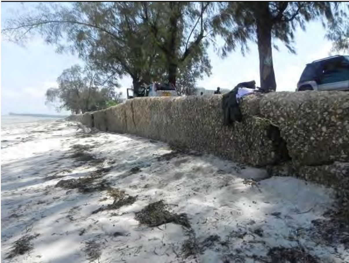
Figure 2-3: Current Situation Of The Sea Wall In Dar Es Salaam To Be Re-Constructed
