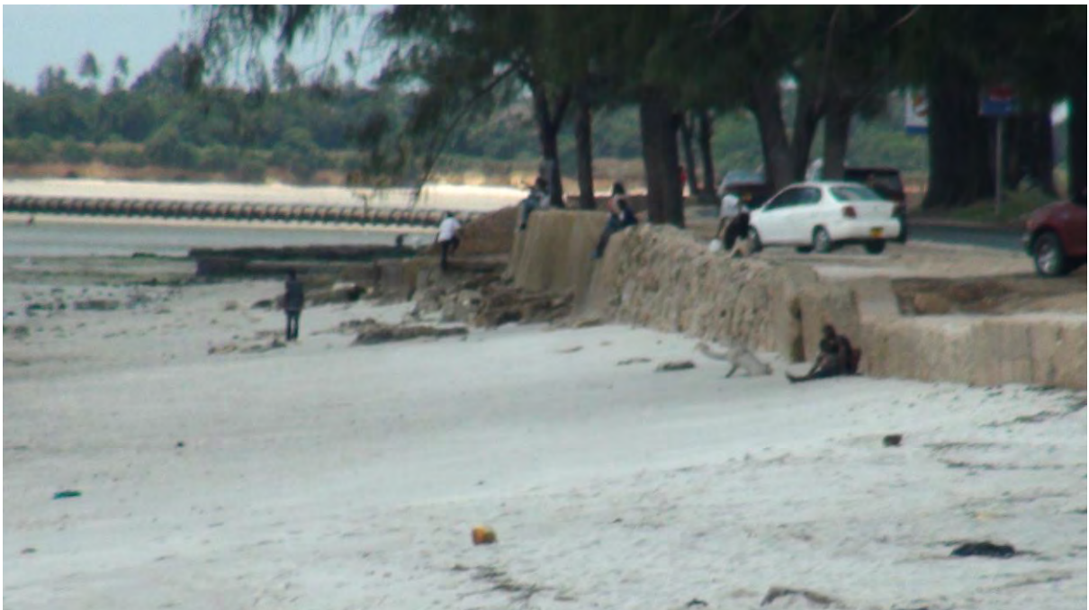
Figures 4-5: Evidence of water movement towards the wall and wall degradation along ocean road.
