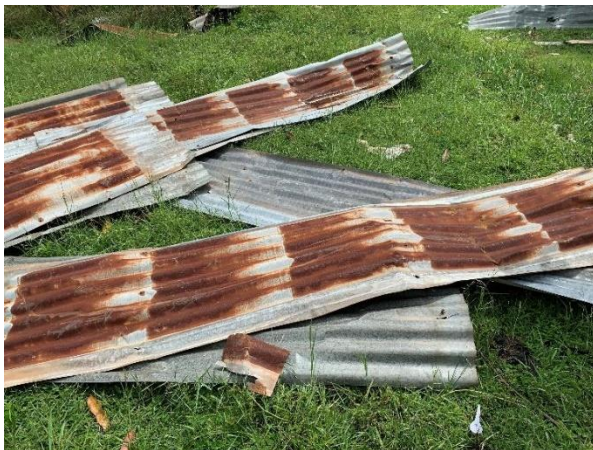
Figure 14 “Damaged corrugated roof sheeting that has been removed from masonry houses due to strong winds.”
