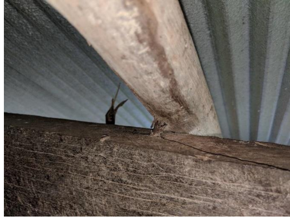
Figure 12 “Example of use of poor materials in local construction. Recurrent failure of critical elements reported as problematic by local populace.”
