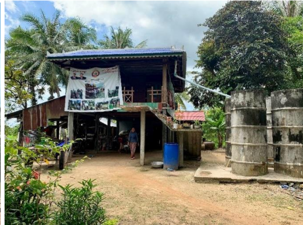
Figure 24 “Typical example of house construction style in flood prone areas.”
