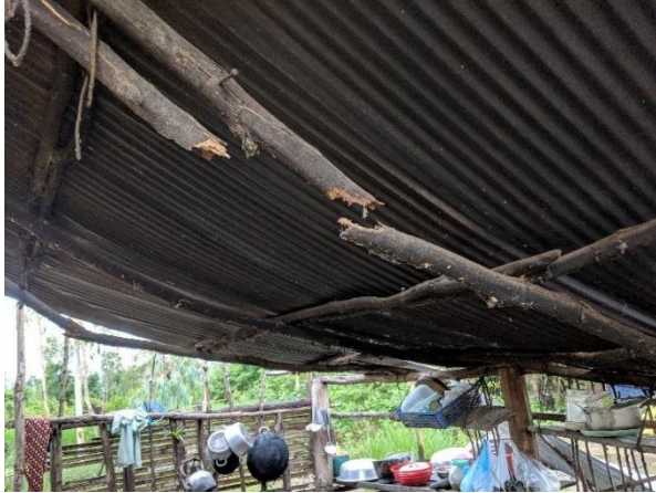
Figure 12 “Example of use of poor materials in local construction. Recurrent failure of critical elements reported as problematic by local populace.”
