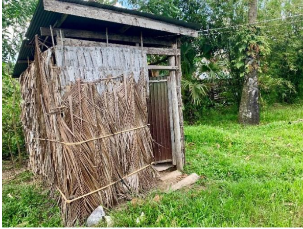
Figure 8 “Typical external latrine construction/ arrangement. According to census data, in many communes, up to 70% of houses did not have their own latrine.”
