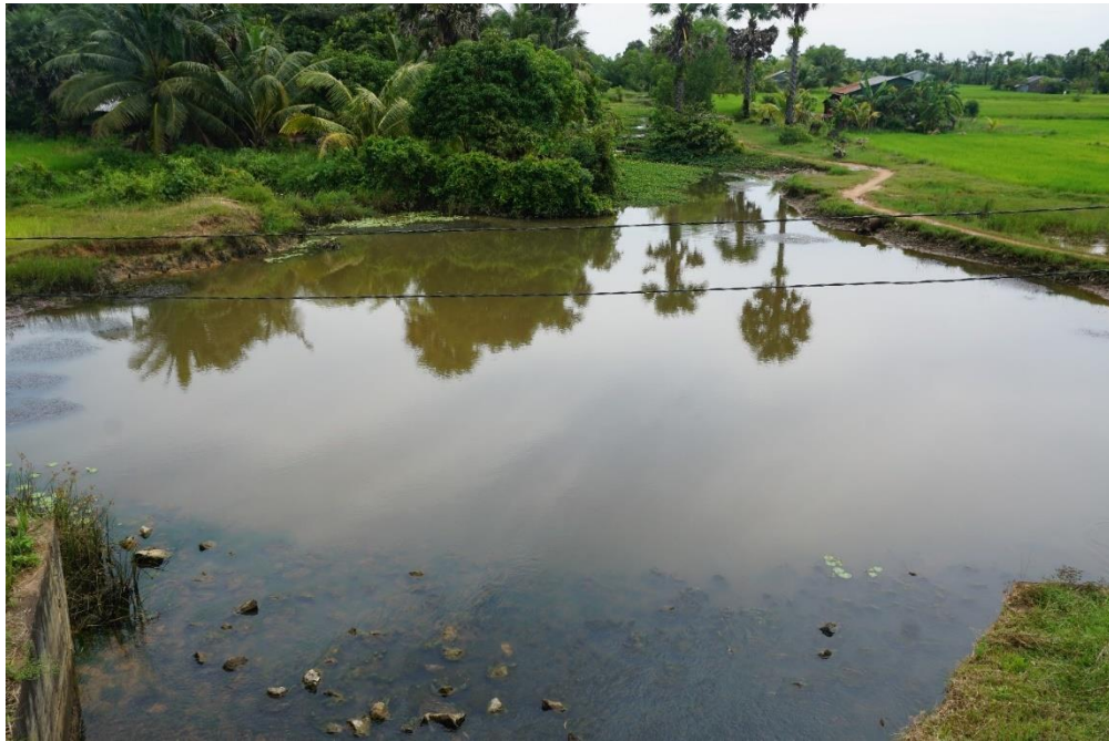
Figure 8 “Silted canal downstream double sluice gate east of O Thmar Reservoir”
