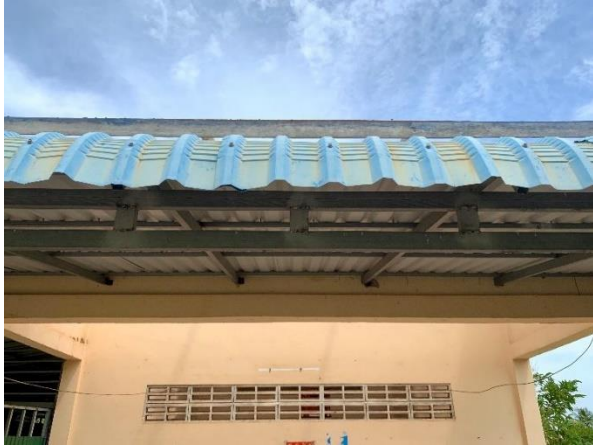
Figure 10 “Example of higher quality corrugated sheeting construction. Use of screws with washers evident. Higher quality corrugated steel noted as composed of thicker material.”
