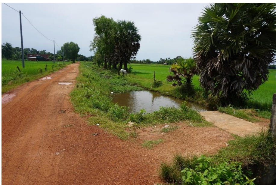
Figure 12 “Canal downstream from water gate 3”
