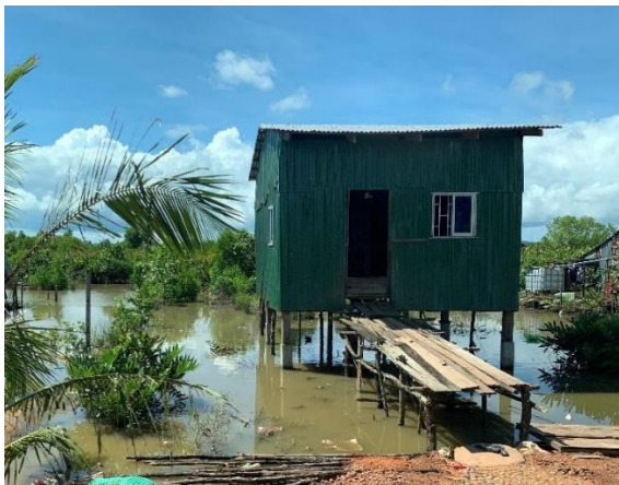
Figure 24 “Typical example of house construction style in flood prone areas.”
