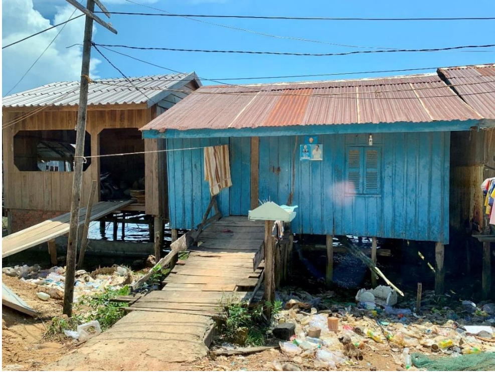
Figure 7 “Typical housing construction for informal settlements along coastline. This house is located in Kep Commune.”
