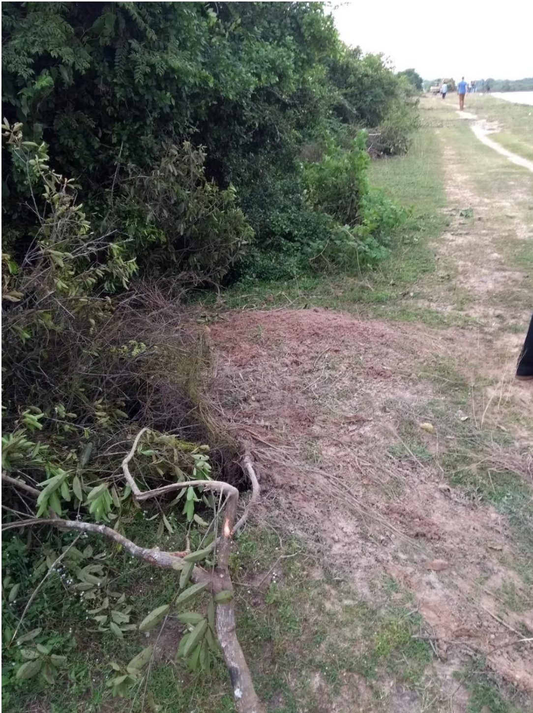
Figure 2 “Downstream face of the dam with dense vegetation and root bole damage.”
