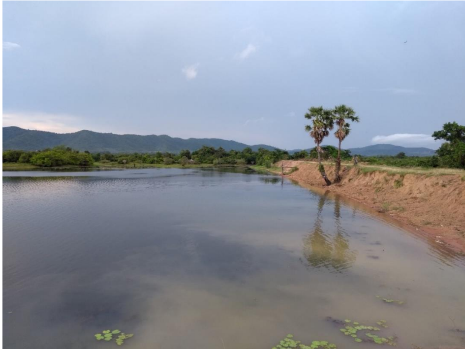
Figure 5 “View along east side of reservoir, showing upstream face with some vegetation.”
