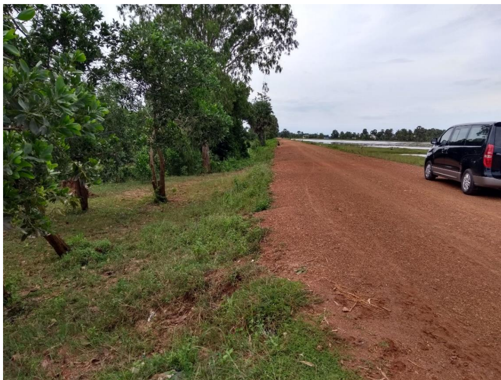
Figure 5 “O Thmar Embankment”
