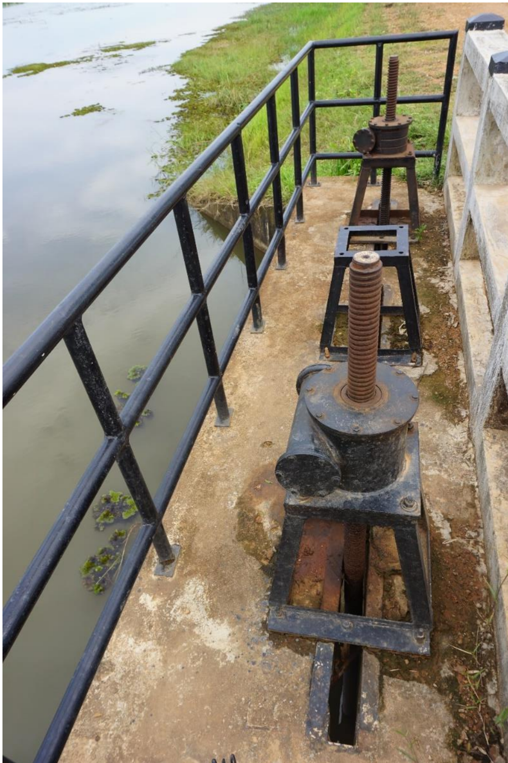
Figure 4 “underpass O Thmar sluice”
