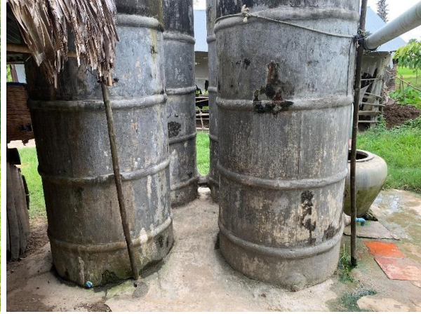
Figure 8 “Typical external latrine construction/ arrangement. According to census data, in many communes, up to 70% of houses did not have their own latrine.”
