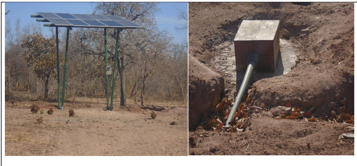
Fig. 31 Pictures of solar powered borehole drilled by ZRBF in Binga Ward 25
