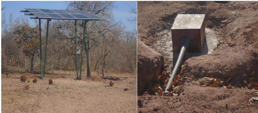
Figure 33 Pictures of solar powered borehole drilled by ZRBF in Binga Ward 25
