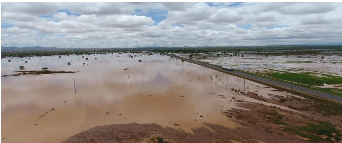
Figure 2: Seasonally flooded Mbuga area where the Dodoma –Dar es Salam road acts as a barrier to drainage.
