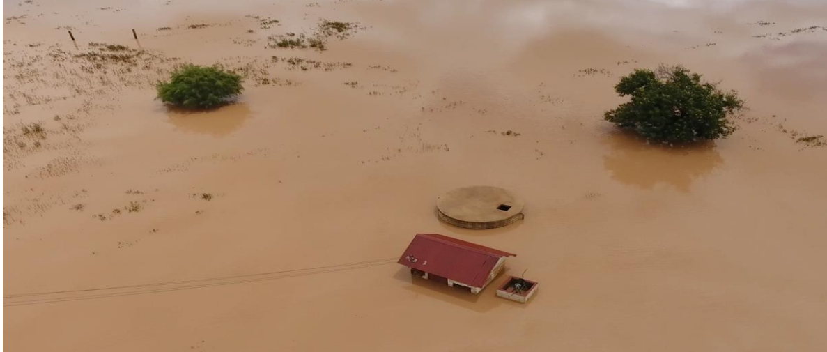
Figure 3: Flooded pump house at Mbuga area in Mtanana village
