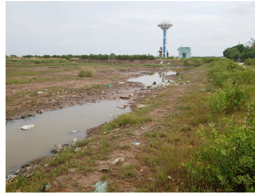
Figure 8. Water tank in the community
