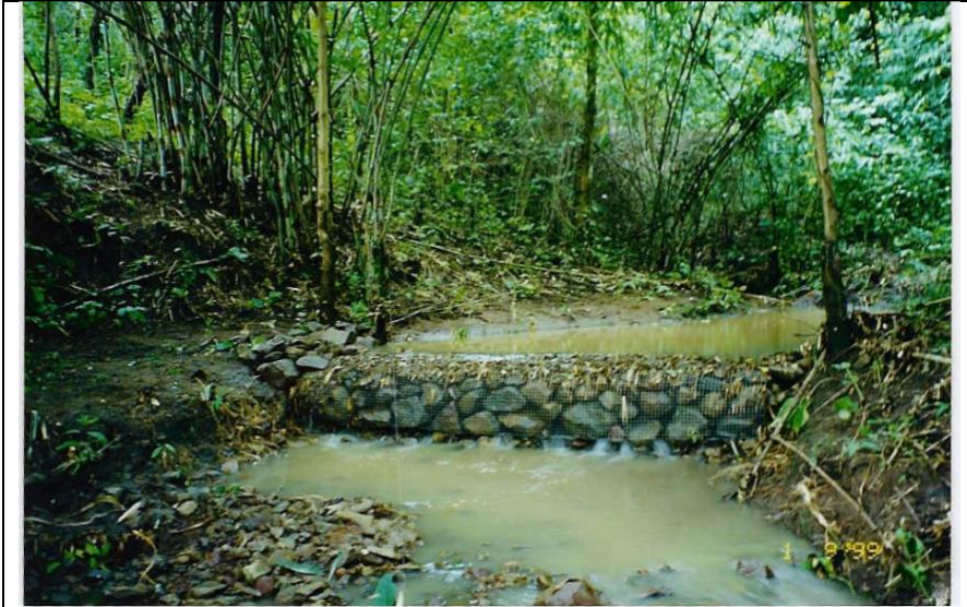
Figure 19: Example of a rehabilitated weir.
