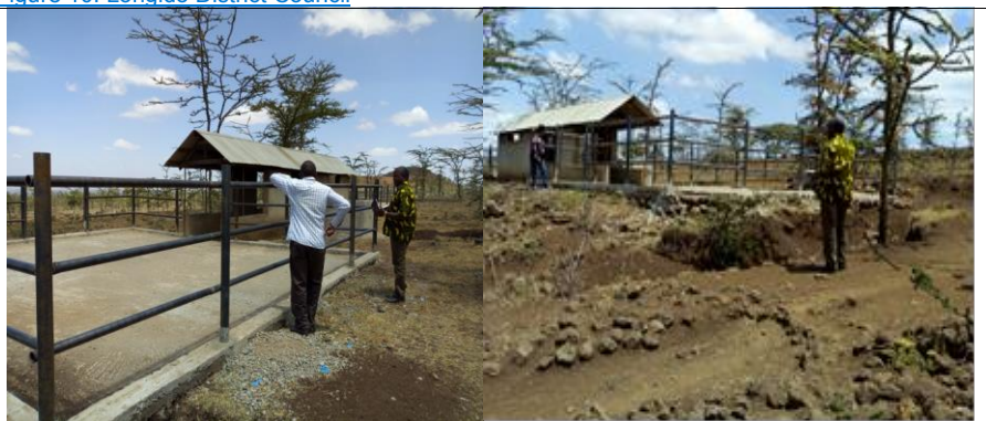
Rehabilitated cattle dip in Lerangwa village.
