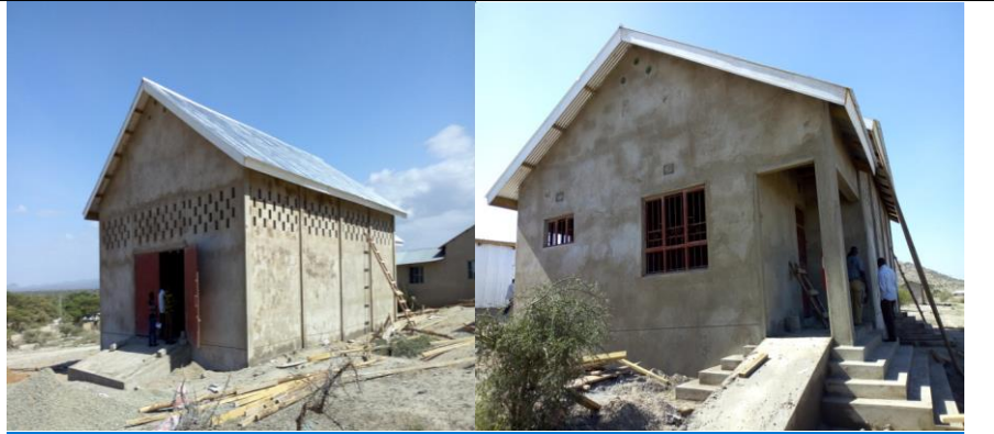
Food storage warehouse at Mairowa ward
