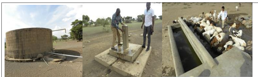
Water storage tank, water delivery points (DPs) and cattle trough in Irendeni Village, Engaruka
