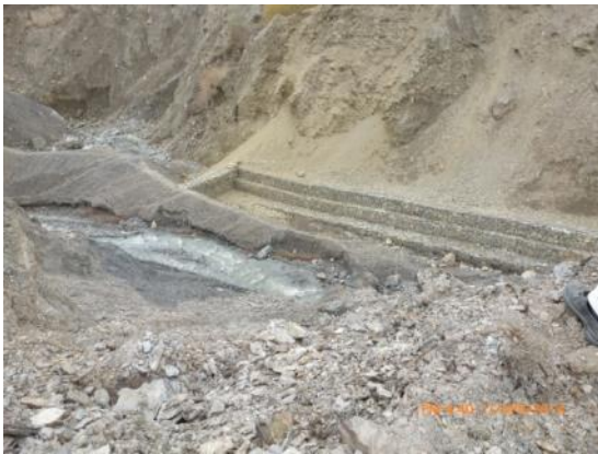
Gabion protection wall and excavated diversion at Ozagh (Gokhir) village
