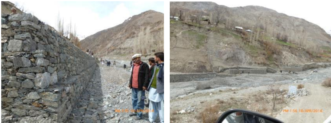
Gabion protection walls at Bindo Rathani (Drongagh)
