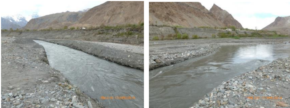
Excavated river channel on the left side and diversion dike on right side for Chitral River at Shogram Payen village Bindo Gole
