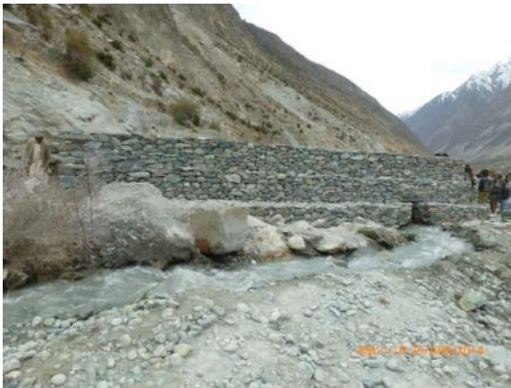
Photo of completed first portion of protection wall at village Chira Bari Bar Bagrote
