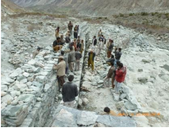
On right side photo of whole protection wall under construction & on left side villagers are busy in construction
