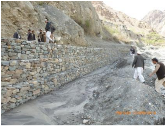
Gabion protection walls at Shogram village
