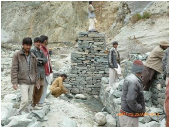
On right side photo of whole protection wall under construction & on left side villagers are busy in construction
