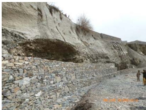
Gabion protection wall and excavated diversion at Ozagh (Gokhir) village
