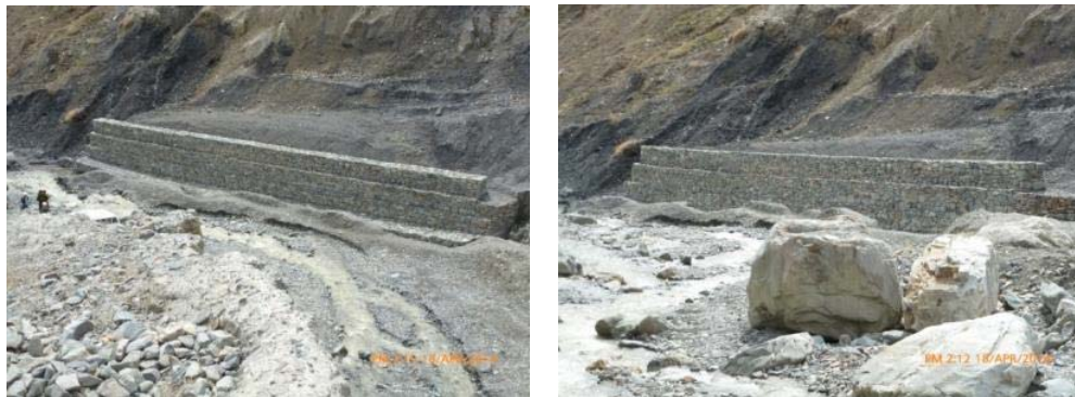
Gabion Protection walls at Gobashedeh (Drongagh).
