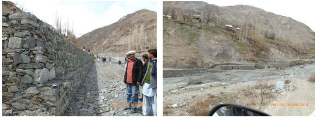
Gabion protection walls at Bindo Rathani (Drongagh)
