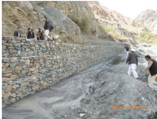
Gabion protection walls at Shogram village
