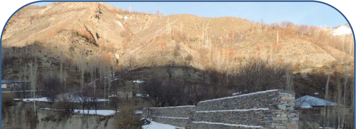
Figure 6 Climate Change Adaptation structures as constructed to reduce the vulnerability of the exposed communities. Note the construction of gabion walls both at the foot slope, aimed at resisting
