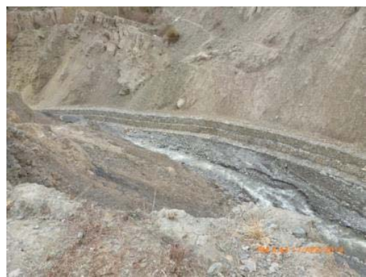
Gabion protection wall and excavated diversion at Ozagh (Gokhir) village
