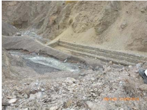
Gabion protection wall and excavated diversion at Ozagh (Gokhir) village
