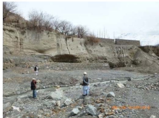
Gabion protection wall and excavated diversion at Ozagh (Gokhir) village
