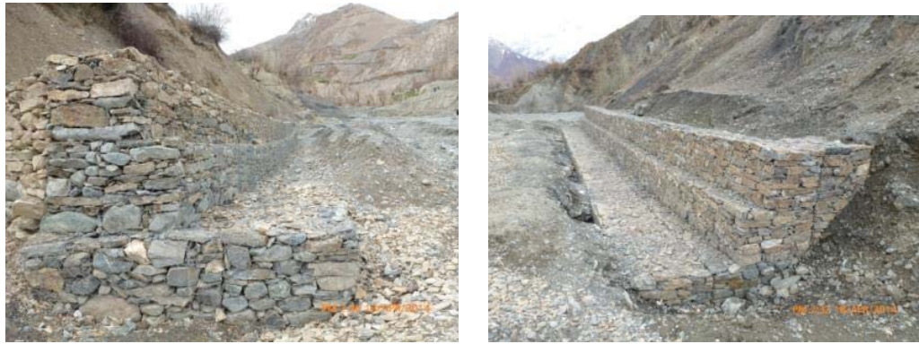
Gabion protection walls at Pongodur (Drongagh)
