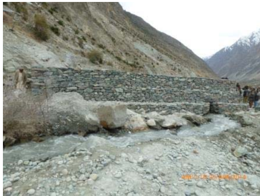
Photo of completed first portion of protection wall at village Chira Bari Bar Bagrote
