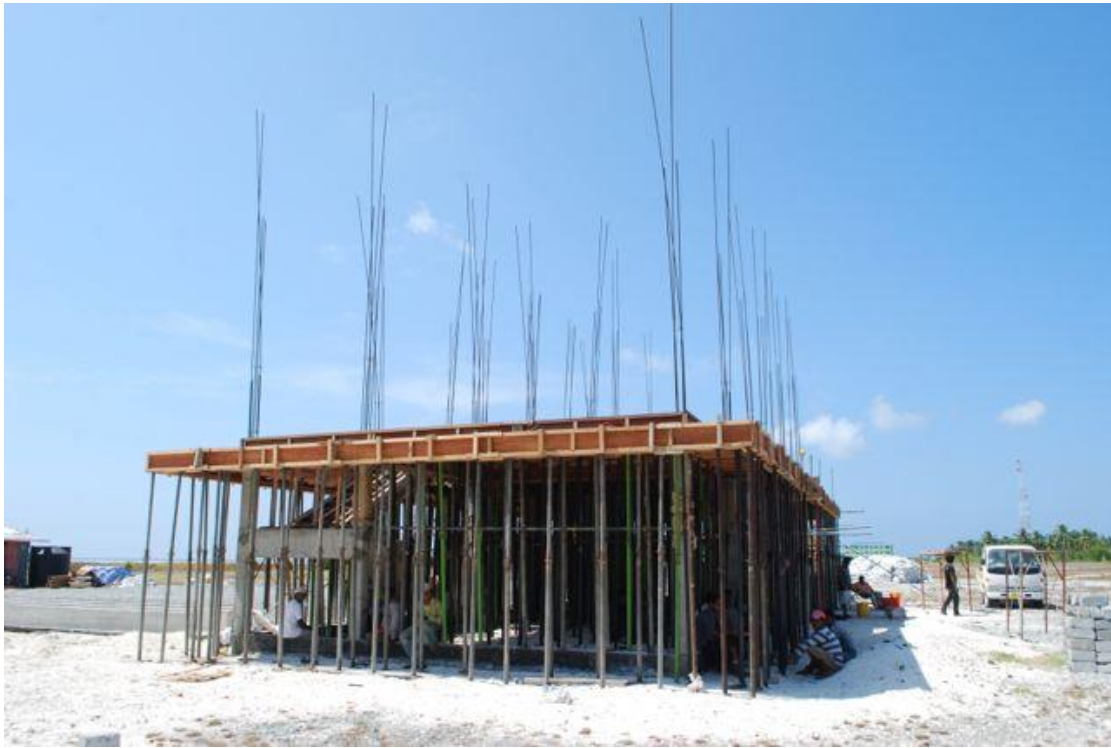
Photo 15 Gadhdhoo RO Plant Building
