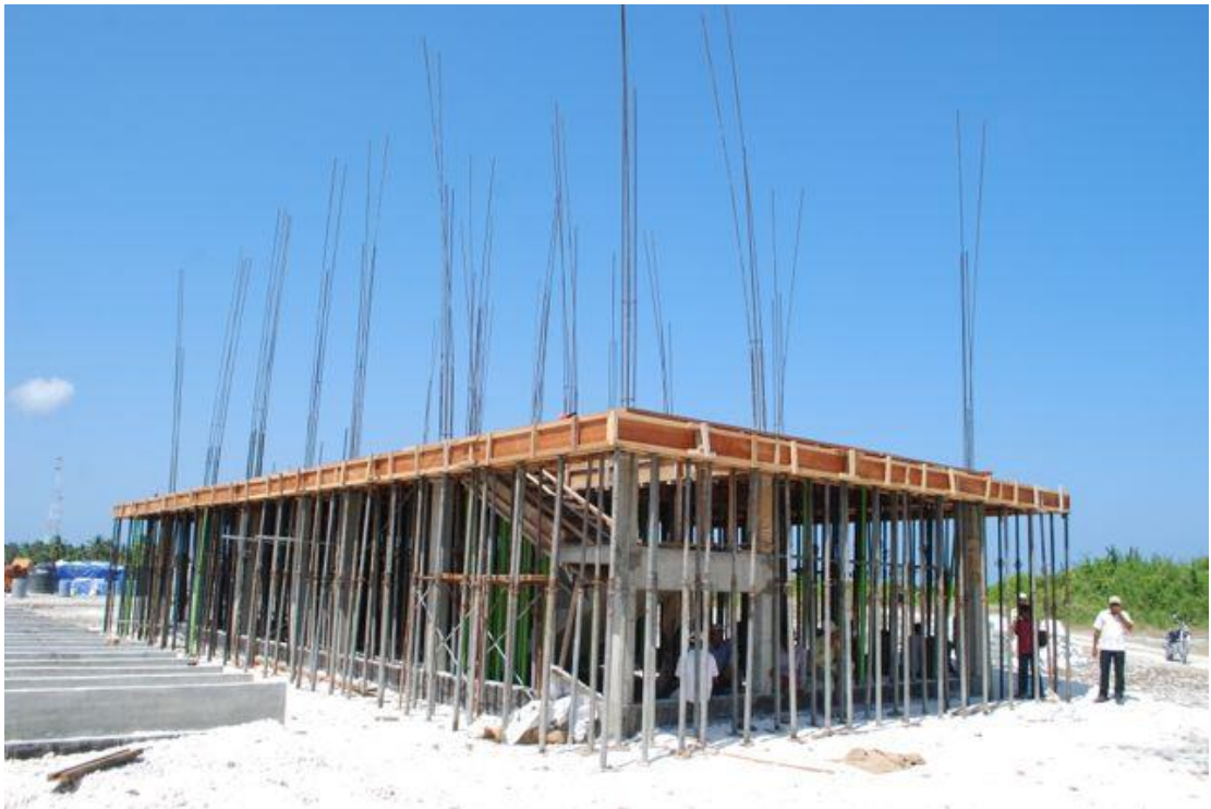
Photo 16 Gadhdhoo RO Plant Building
