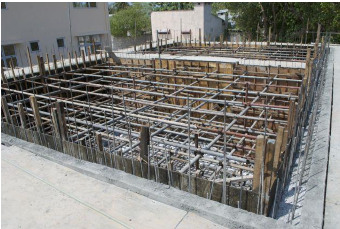
Photo 6 Mahibadhoo Rainwater Collection Tank 1 (top)
