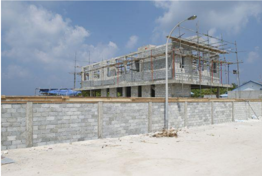
Photo 9 Mahibadhoo RO Plant Building
