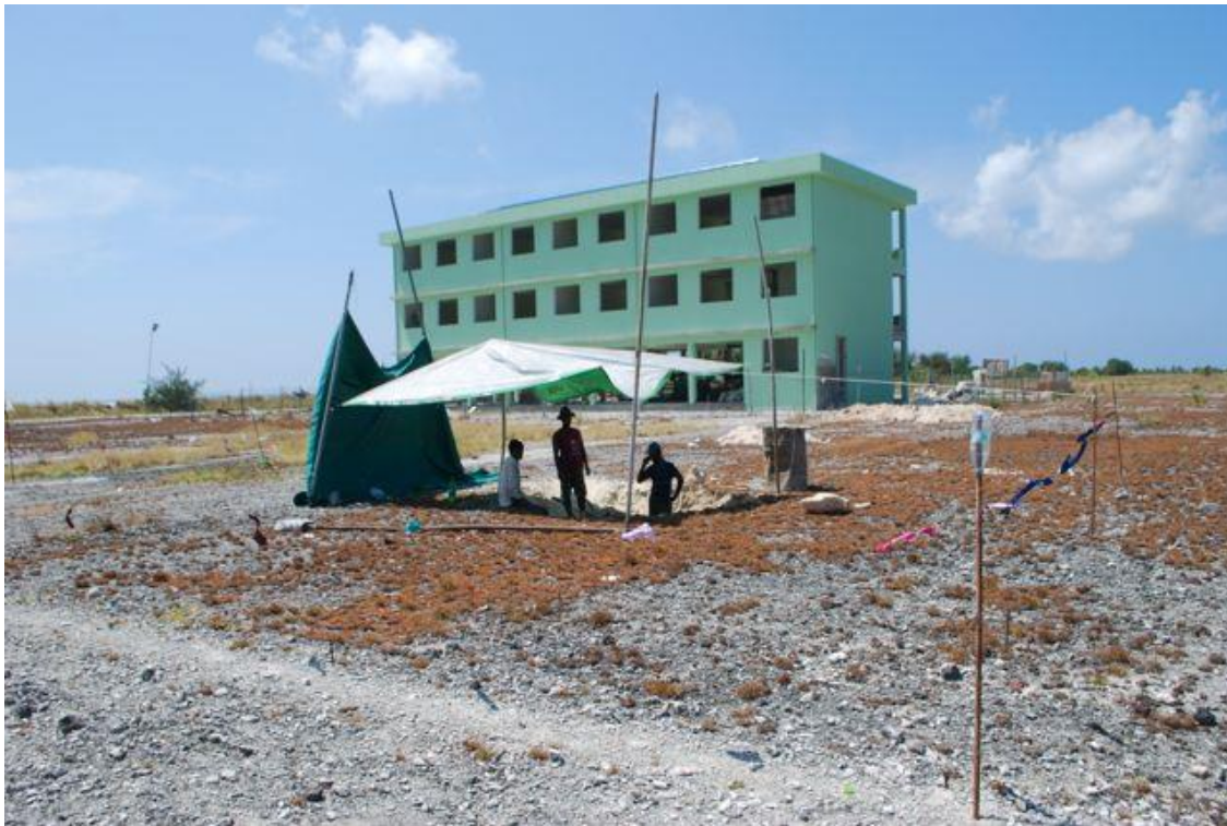
Photo 14 Gadhdhoo Rainwater Collection Tank 1 (site)
