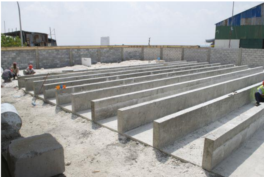
Photo 4 Mahibadhoo GRP Tank Foundation
