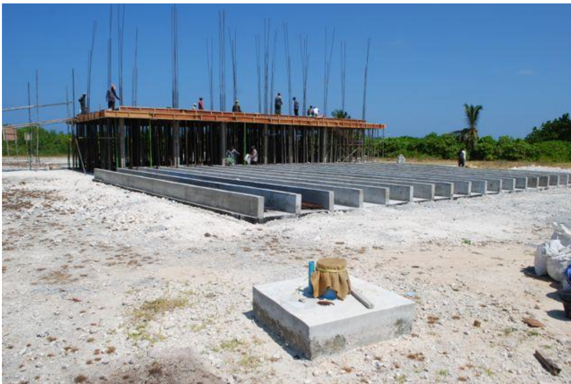
Photo 18 Gadhdhoo RO Plant Building, GRP Tank Foundation, and Borehole
