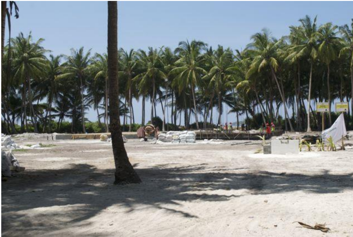
Photo 3 Ihavandhoo RO Plant Site
