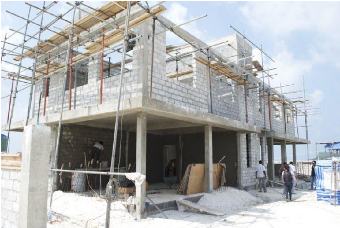
Photo 10 Mahibadhoo RO Plant Building
