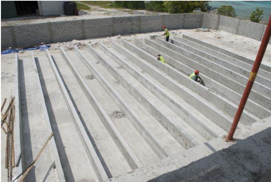
Photo 5 Mahibadhoo GRP Tank Foundation
