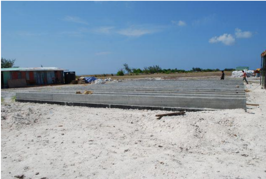
Photo 13 Gadhdhoo GRP Tank Foundation
