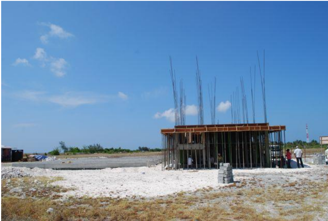
Photo 17 Gadhdhoo RO Plant Building and GRP Tank Foundation
