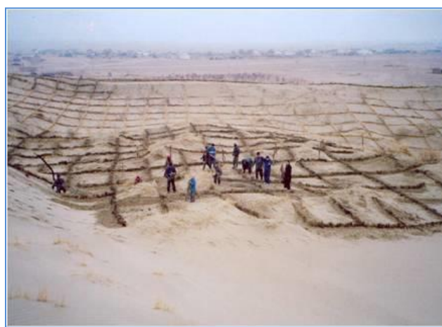
Dune fixation with reed cells in desert region of Garagum
