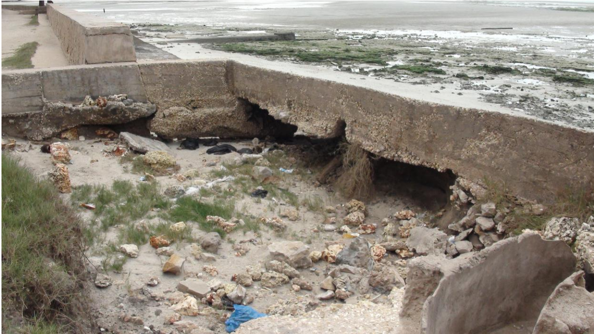
Figure 7: Evidence of severe degradation in sea wall along Ocean road.
