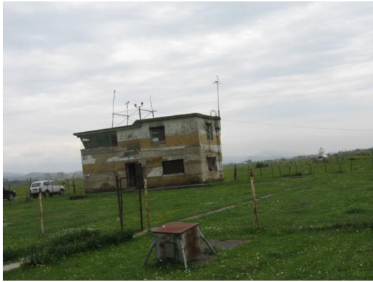
e) Hydrometric Station building station
