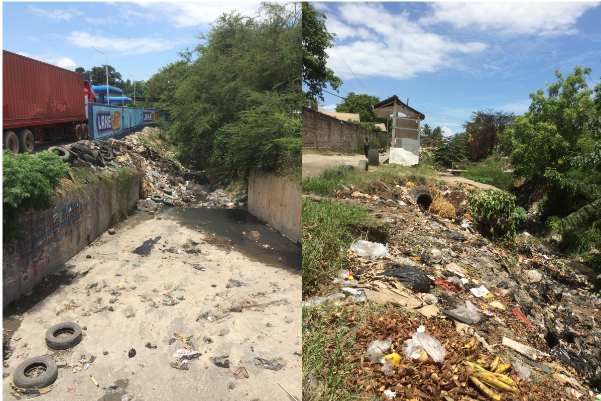
Photo 2: Importance of solid waste management in the rehabilitation of drainage systems in Dar es Salaam
