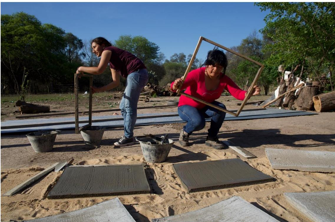
Picture2: Women producers working in the construction of cement tile-roof cisterns, province of Chaco
