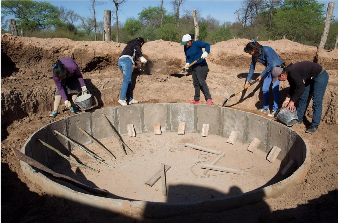
Picture1: Women producers working in the construction of cement tile-roof cisterns, province of Chaco
