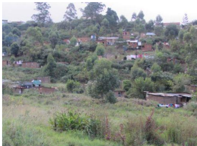
Figure 3: Informal settlement located on floodplain and adjacent steep slopes
