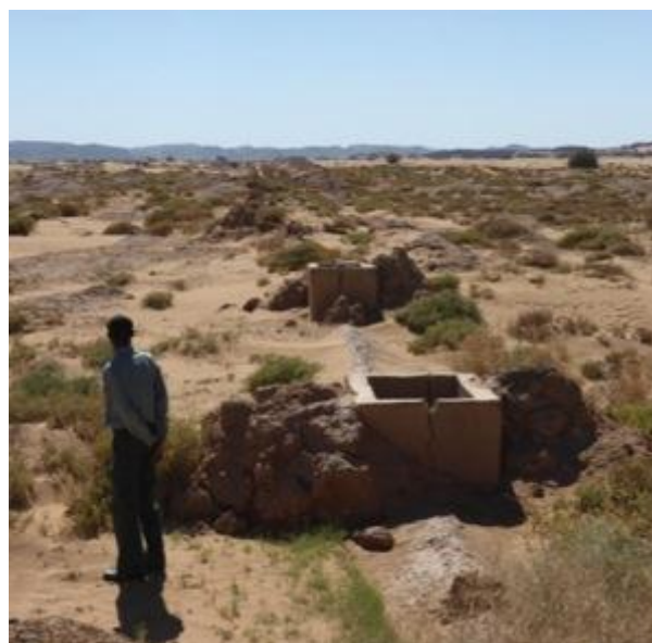
Figure 17 : Partially restored Khettara in Bouya
