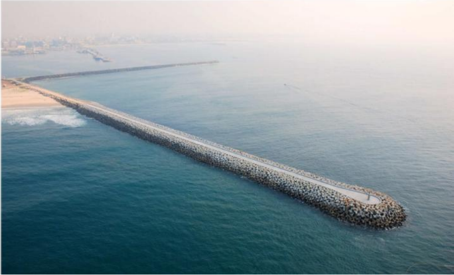
Figure 1.5 : Sand stoppage groyne at the Port of Cotonou extended of 300 in 2010.
