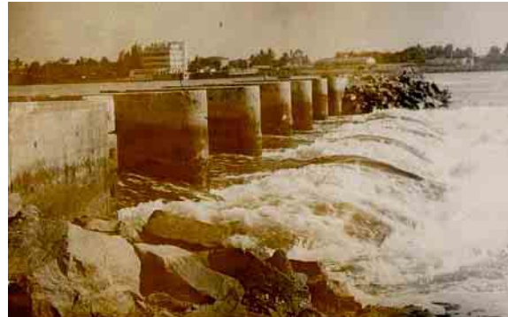
Figure 2.3 : Sluice dams at Cotonou channel mouth
