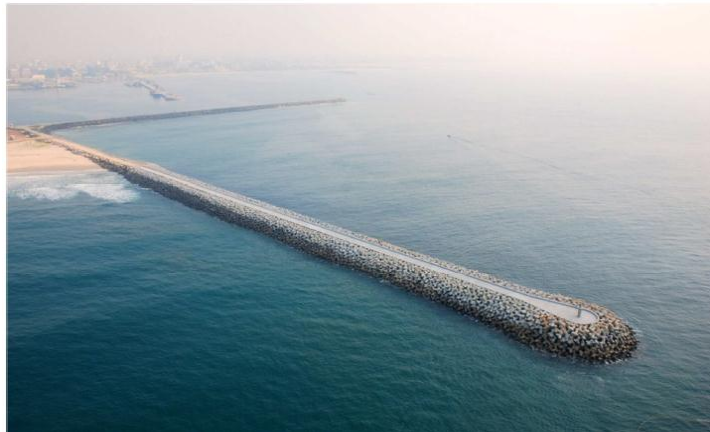
Diagram 1.12 : Sand stopping groyne at the Cotonou sea port prolonged to 300 in 2010.
