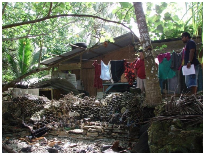
A self-built gabion (metal frame filled with rocks) in Malem: Photo: Iris Monnereau
