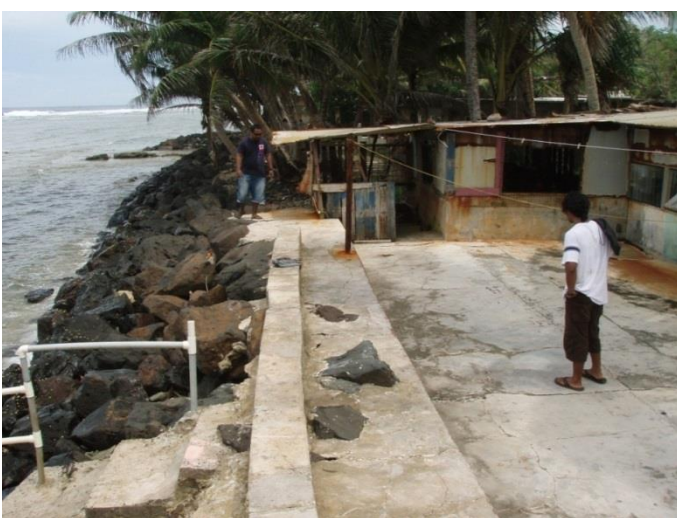
The seawall behind the house and bakery of Kilafwasru Kilafwasru and Sepe Kilafwasru in Malem (box 4.5). Photo: Iris Monnereau
