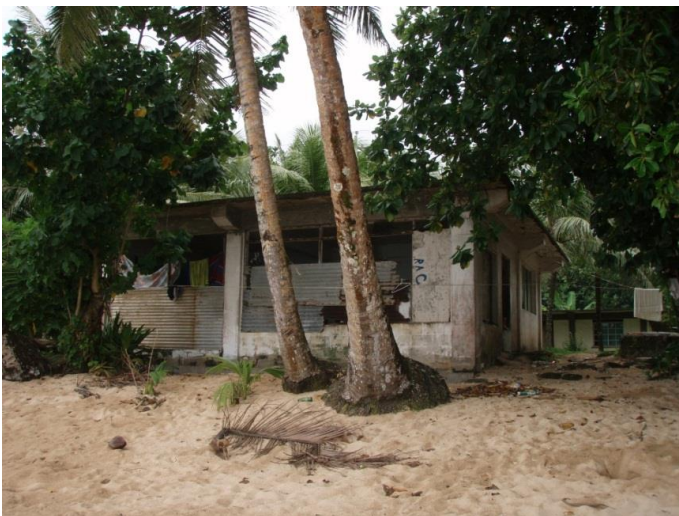
The destroyed house of Sepe Santos (box 5.3). Photo: Iris Monnereau
