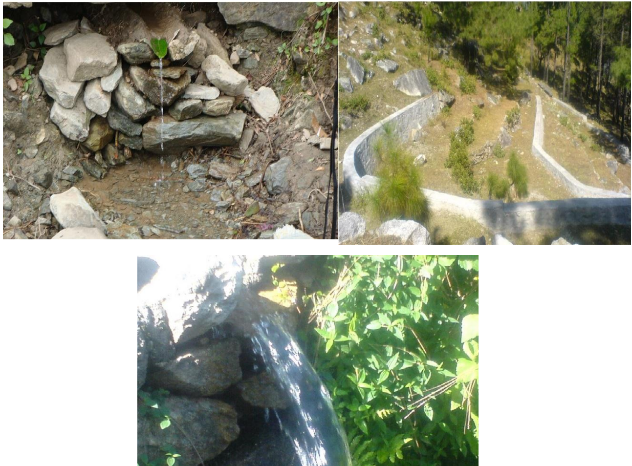
Figure 9: Photographs of Spring Rejuvenation done by BARC in Uttarakhand a. Drying Spring b. Water recharge through constructing water harvesting structures c. Rejuvenated Spring
