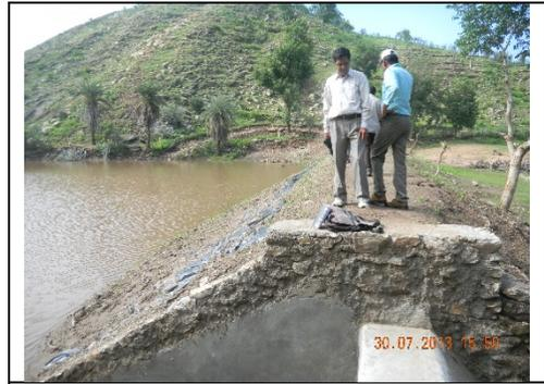
*LDPE lining in earthen embankment structure*
