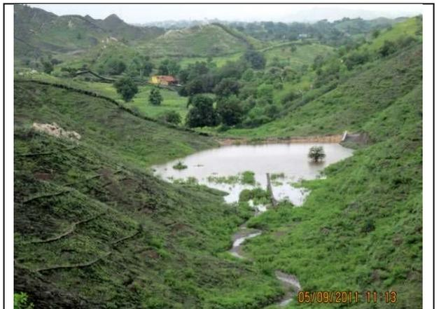
*An earthen embankment with spillway*
