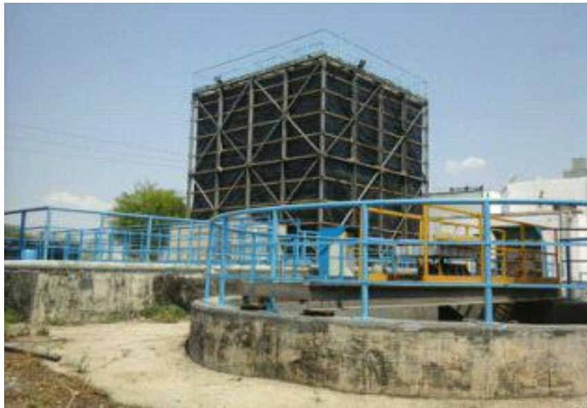
FIGURE 9: VIEW OF THE WWTP AT TAL MANTAH
