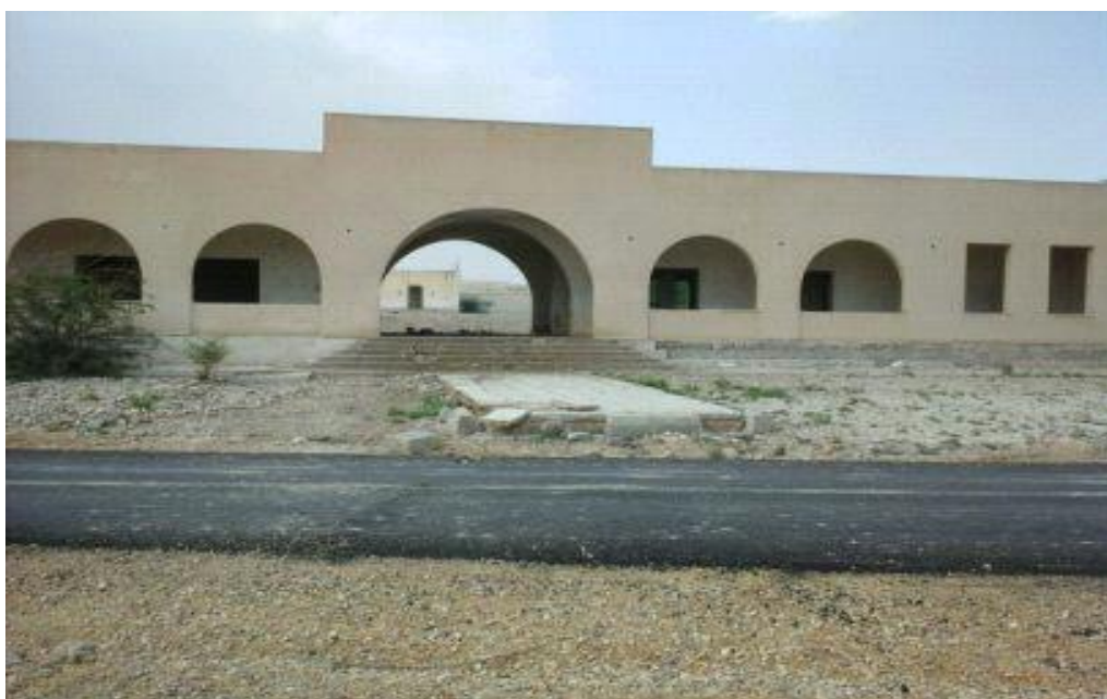
FIGURE 12: WUA/ VISITOR KNOWLEDGE CENTRE TO BE REHABILITATED
