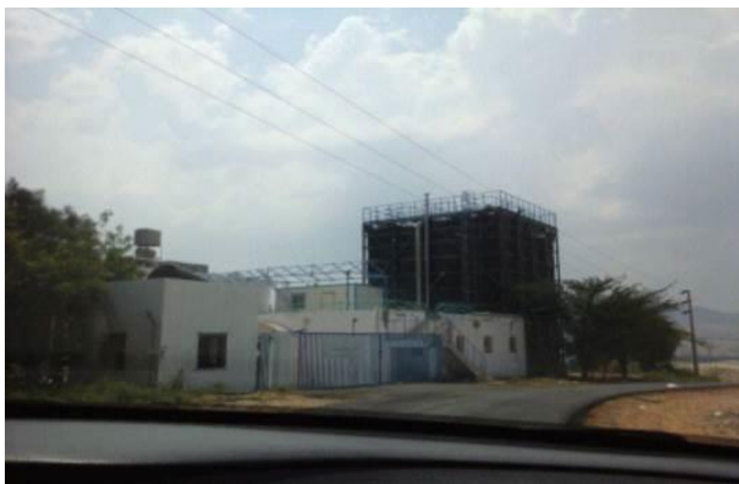
FIGURE 8: THE TAL MANTAH WWTP
