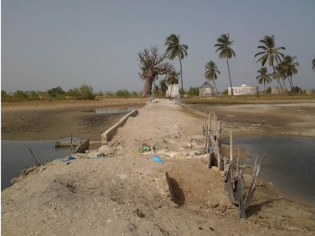
Figure 2: Dike protecting against rising sea water built by populations in Colbassy (CSE, January 2015)
