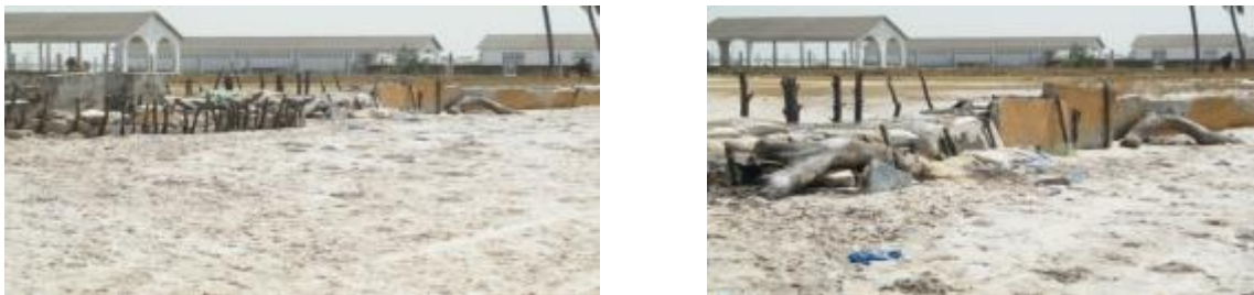
Picture 2: Dike located in front of the village
