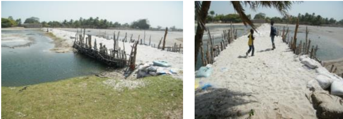
Picture 1: Ndioundiouré dike
