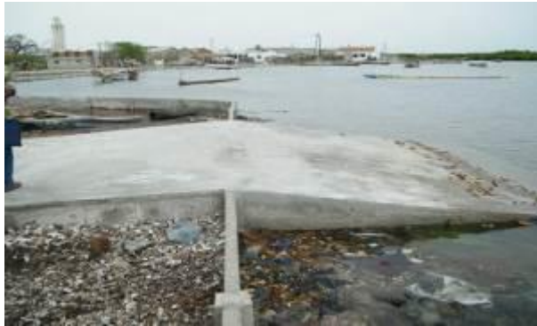
Photo 14: Dike made of RC plates
