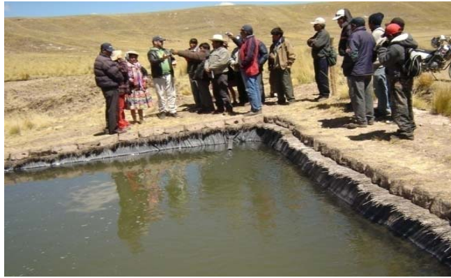
Photo: Type of earthen dyke to be constructed for the storage of snowmelt and from the short rainy season. Source: COPASA Archives (2012). The image corresponds to dykes operating in the region
