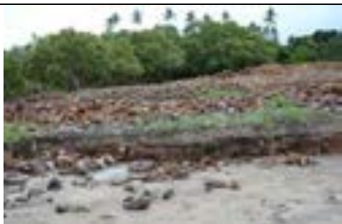
GPS 11 5° 25' 39.486" S; 38° 58' 3.698" E Figure 10: Flanking effect alongside southern Pangani seawall
