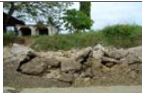
GPS 216 6° 9' 26.118" S; 39° 12' 3.946" E Figure 6: Crumbling and collapse of Bwawani seawall
