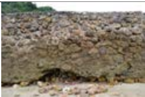
GPS 80 5° 25' 56.071" S; 38° 58' 27.944" E Figure 5: Scour on northern seawall
