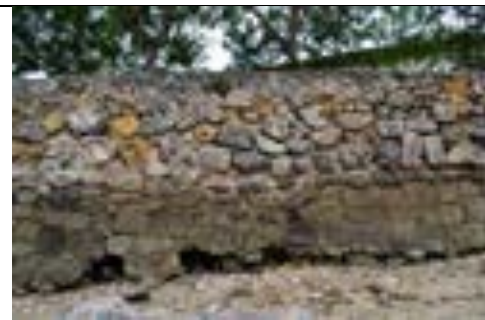
GPS 87 5° 25' 54.430" S; 38° 58' 22.307" E Figure 6: Scour northern seawall
