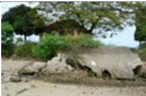
GPS 215 6° 9' 26.255" S; 39° 12' 4.097" E Figure 5: Crumbling and collapse of Bwawani seawall
