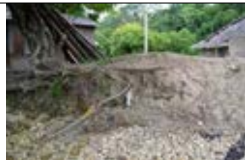
GPS 102 5° 25' 55.222" S; 38° 58' 16.288" E Figure 12: Flanking effect alongside northern Pangani seawall in Bweni village 160
