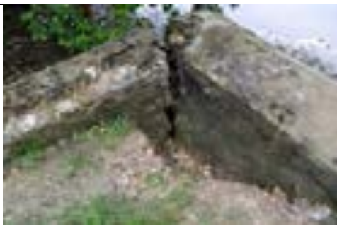
GPS 30 5° 25' 43.550" S; 38° 58' 16.630" E Figure 8: Cracking and landward erosion along southern seawall
