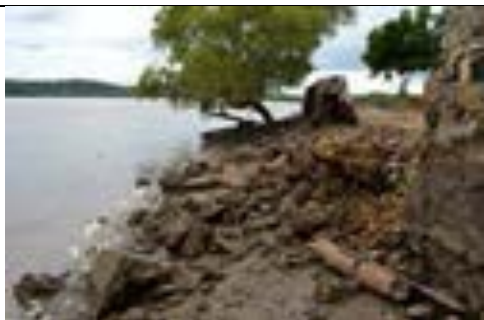
GPS 20 5° 25' 42.643" S; 38° 58' 9.995" E Beginning of gap, GPS 21 end of gap Figure 7: Collapse along southern seawall
