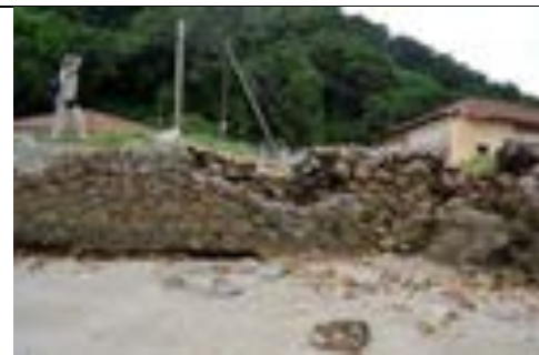
GPS 79 5° 25' 56.280" S; 38° 58' 28.286" E Figure 9: Collapse along northern seawall
