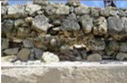
GPS 467 6° 48' 35.280" S; 39° 17' 50.262" E (2.4h X 1.2w) Figure 13 Erosion above concrete step 0.9m in.
