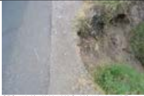
GPS 459 6° 48' 36.788" S; 39° 17' 51.547" E Figure 8: Circled in Figure 7: tarmac of Ocean Road and erosion
