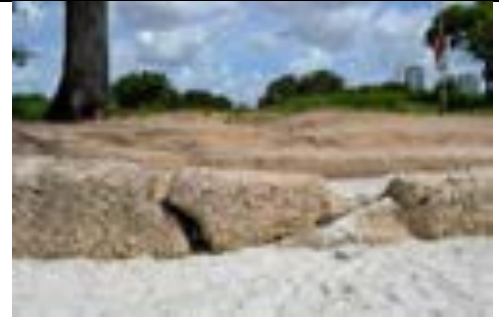
GPS 497 6° 48' 22.205" S; 39° 17' 34.026" E (0.45h X 0.75w) Crumbling and portion collapsed Figure 24
