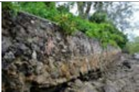
GPS 22 5° 25' 43.079" S; 38° 58' 11.402" E Figure 4: Scour on southern seawall
