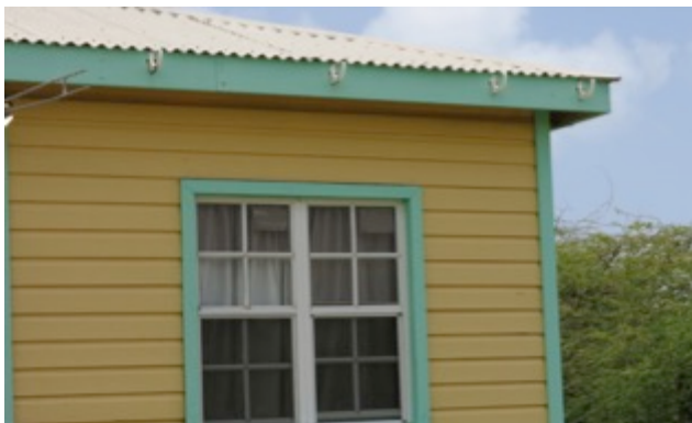
Figure 7. A household in McKinnon’s pond area with braces for rainwater harvesting but no guttering (toilets, sinks, shower heads, installed)
