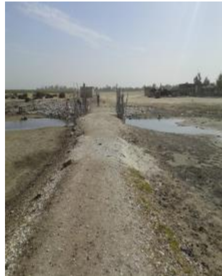
Picture 8: Ndiar dike equipped with discharge nozzles
