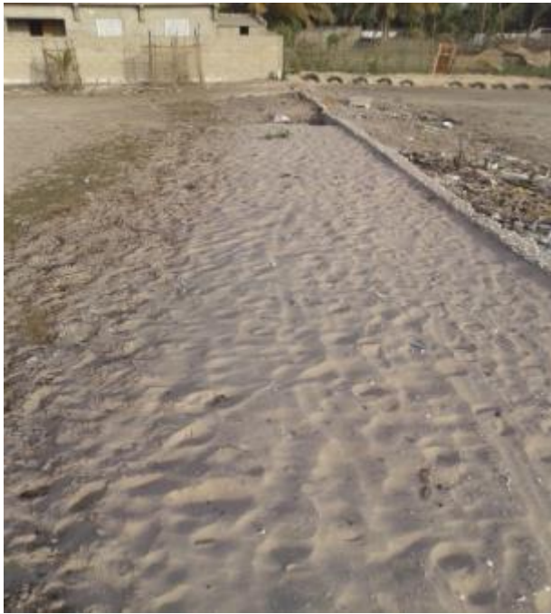
Picture 9: Ndioundiouré dike made up with shell wall, left bank
