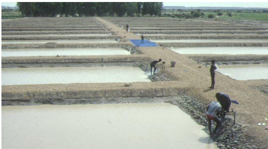
Photo 12: Ponds surrounded by dikes
