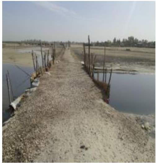
Picture 7: Ndiar dike with a shell embankment
