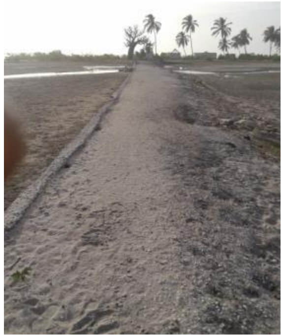
Picture 9: Ndioundiouré dike made up with shell wall, left bank
