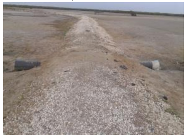
Picture 11 : Ecole 2 dike in damaged shell embankment, left bank
