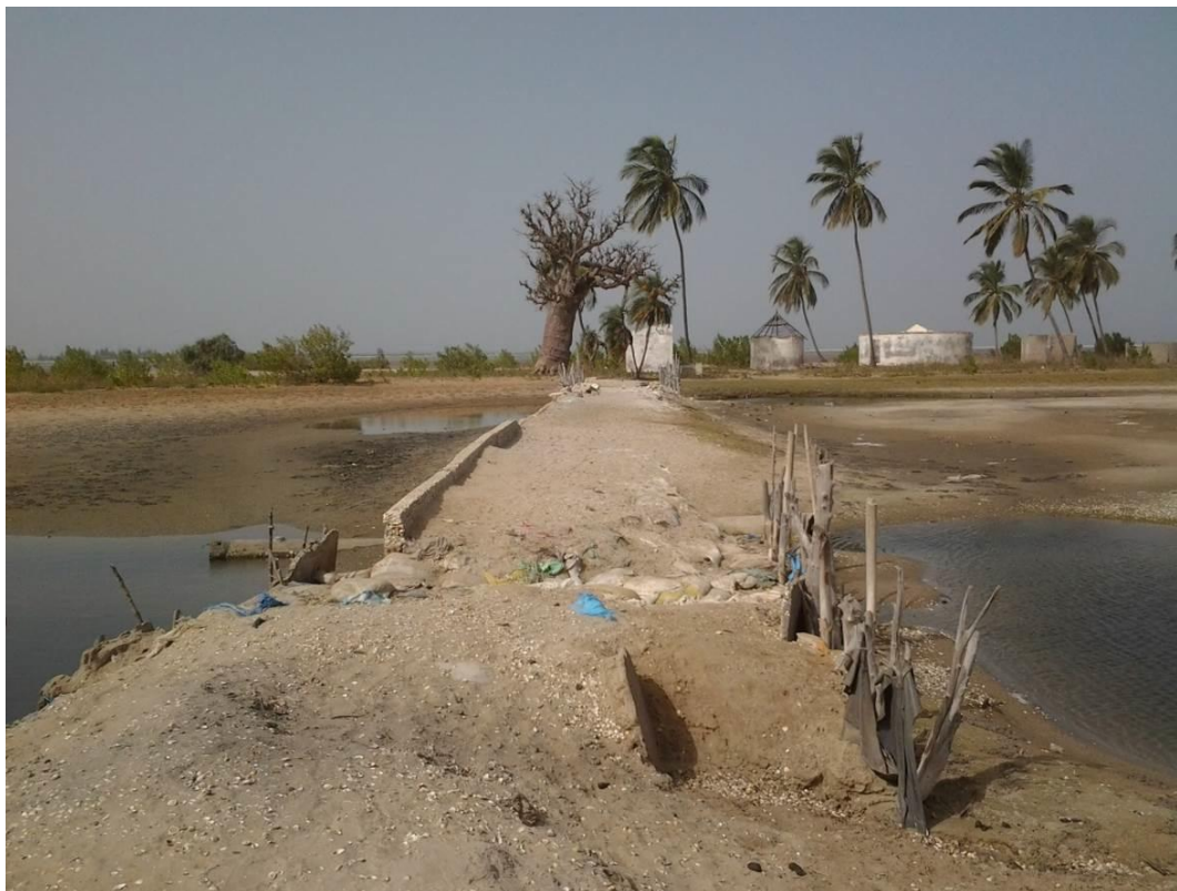
Figure 9: Dike protecting against rising sea water built by populations in Colbassy (CSE, January 2015)
