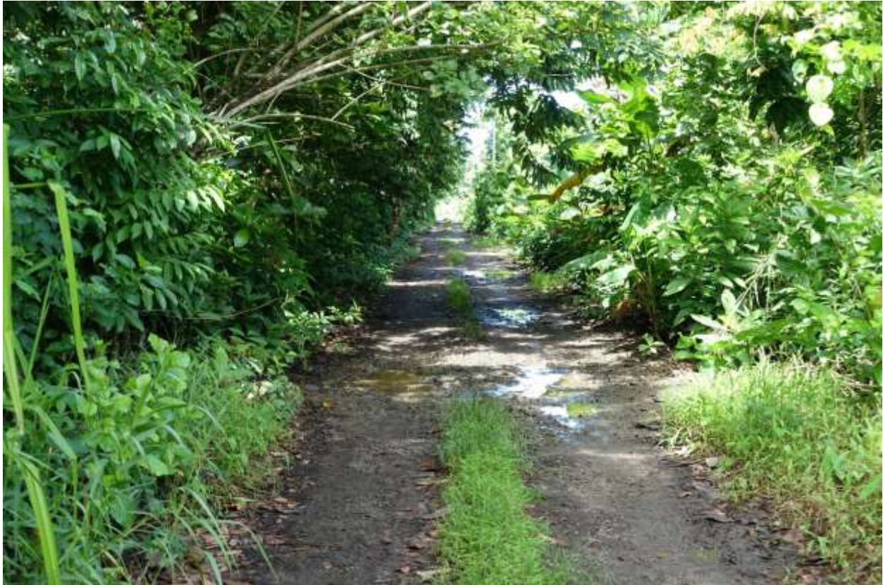
Figure 13: Typical farm road which will be widened and upgraded to a sub-base standard by the project.
