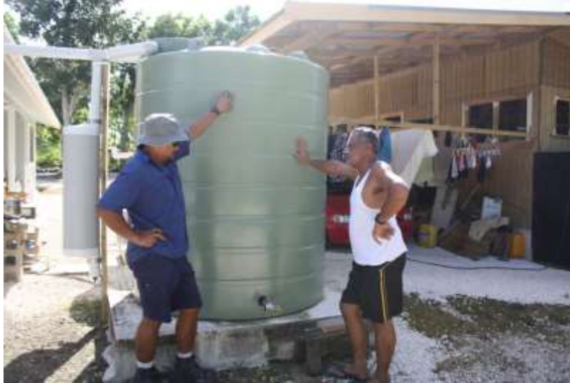
Figure 7. A fully installed rainwater harvesting & storage system (source: PACC Niue, 2014)
