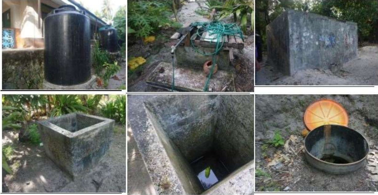
Figure 5 Sample of water tanks and wells from outer islands – Eauripik, Woleai atoll, Ifalik, and Feraulap atoll (Source: Rapid Needs Assessment, March 2016, Yap, FSM)
