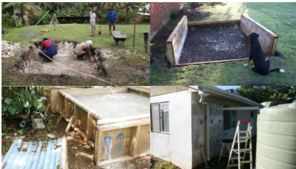
Figure 6 Installing a rainwater harvesting system at the household level (source, PACC Niue,2014)
