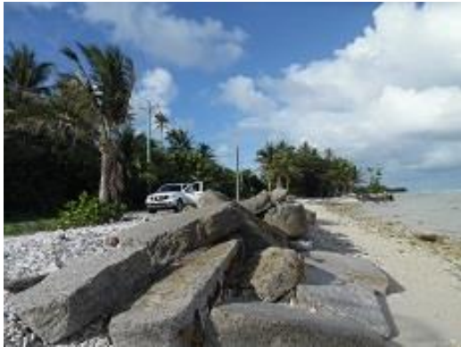
Image 2 Road exposed to over wash
