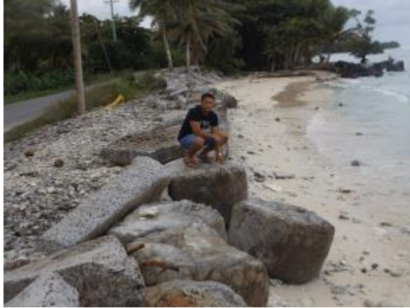
Paal section of malem road. mass concrete bags, loose boulders and broken concrete, placed randomly to reduce surge impact and prevent wave overtopping and erosion of road (photo credit: Simpson Abraham, 2015)
