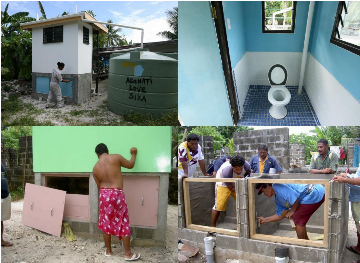
Figure 9 Images of self-composting systems in the Pacific. L-R, a SCT using the roof as a catchment area for rainwater harvesting in Tuvalu (source: IWRM, Nauru). The toilet room, completed SCT in Tuvalu (IWRM, Nauru); construction of chambers, IWP Samoa and Vanuatu
