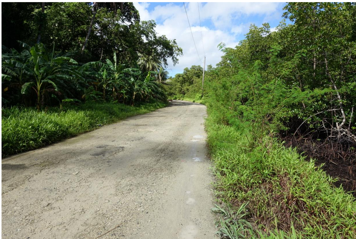
Figure 6: PACC road in Tafunsak completed to sub-base surface standard.
