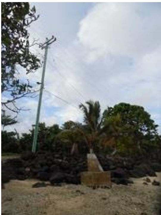
Image 4 Power utilities propped up on nearby shoreline
