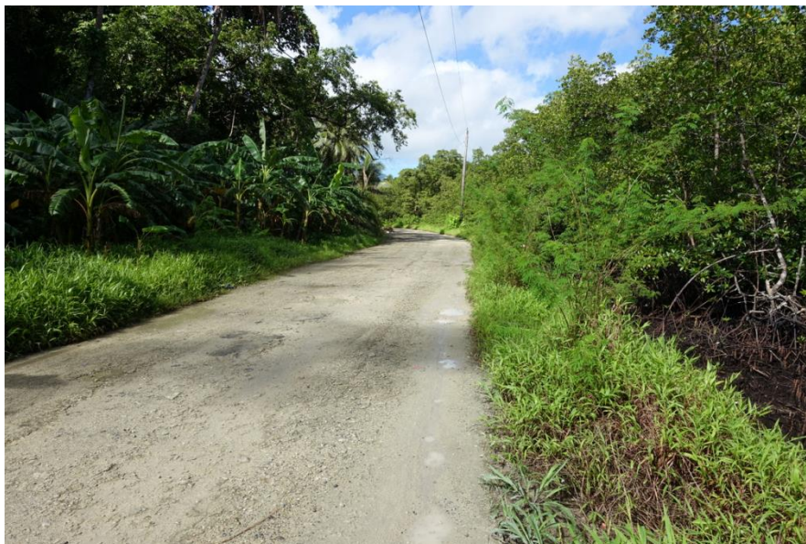
Figure 14: PACC road in Tafunsak completed to sub-base surface standard.
