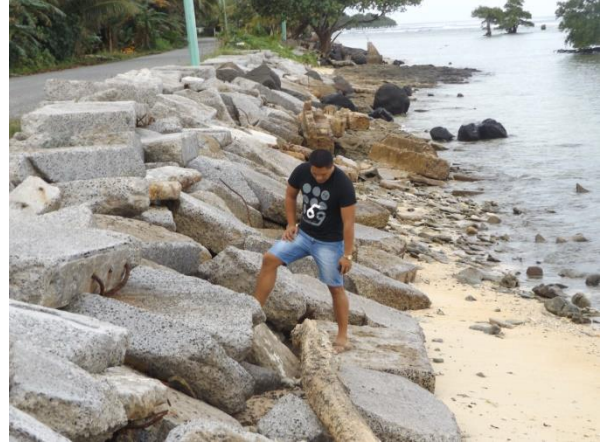
Mosrael section of the coastal road. Existing dumped concrete rubble. A low reef flat breakwater to 'stabilize' shoreline will also be required further south to prevent outflanking and downdrift erosion. (photo credit: Simpson Abraham, 2015)
