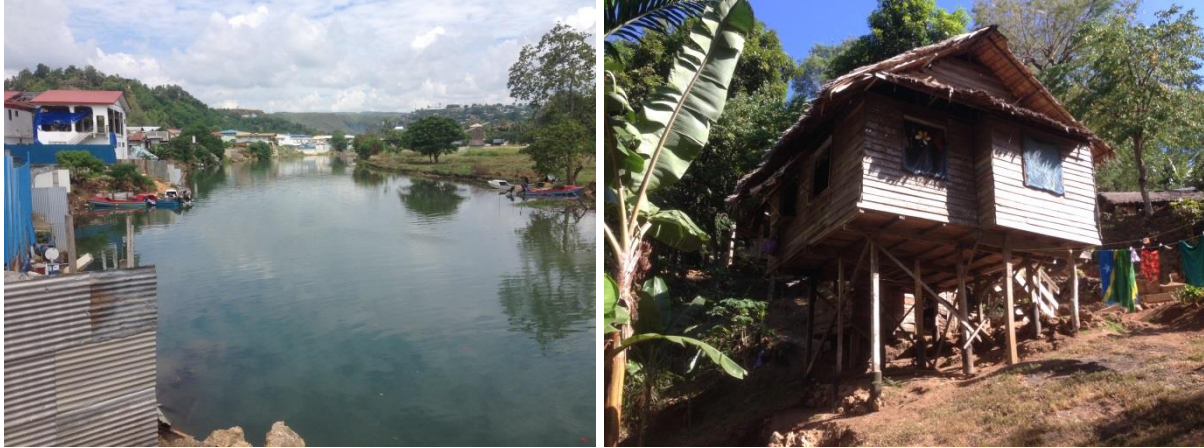
Figure 9: Housing exposed to climate-related risks in Honiara
