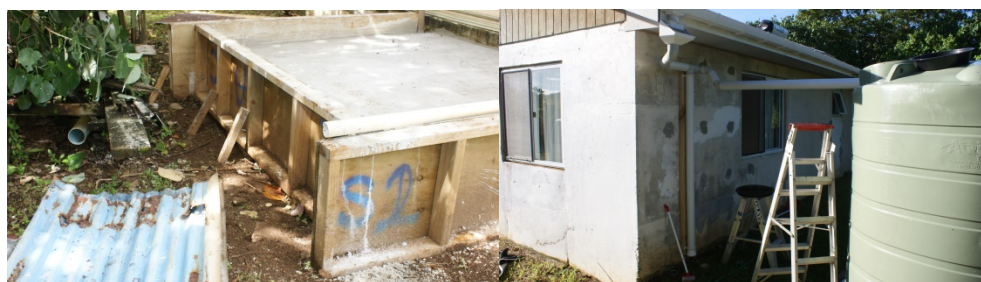
Figure 6 Installing a rainwater harvesting system at the household level (source, PACC Niue,2014)
