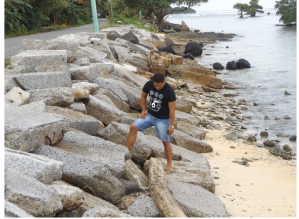
Paal section of the coastal road. Existing dumped concrete rubble. A low reef flat breakwater to 'stabilize' shoreline will also be also be required further south to prevent outflanking and downdrift erosion. (photo credit: Simpson Abraham, 2015)
