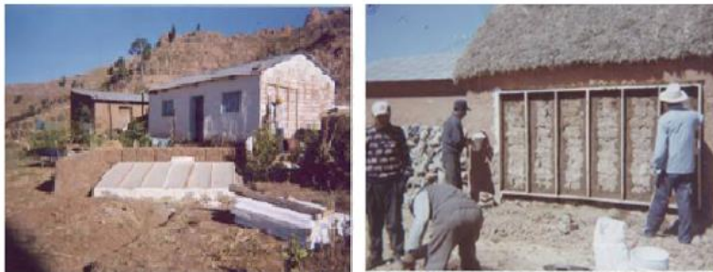
FotoPhoto: Implementation of heaters and Trombe walls, low-cost, accessible technologies. Source: COPASA Archives
