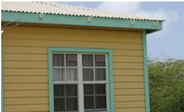
Figure 7. A household in McKinnon’s pond area with braces for rainwater harvesting but no guttering installed
