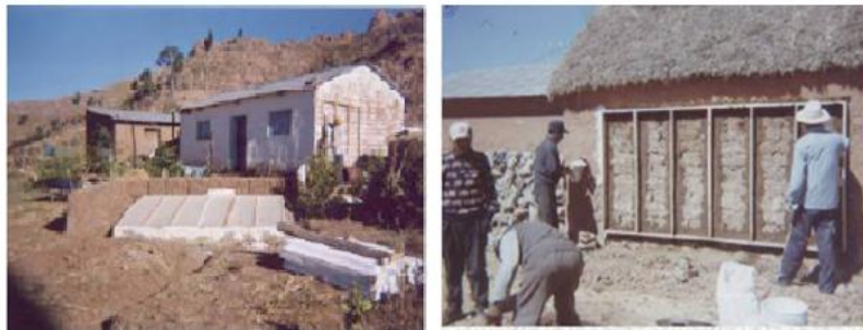
FotoPhoto: Implementation of heaters and Trombe walls, low-cost, accessible technologies. Source: COPASA Archives
