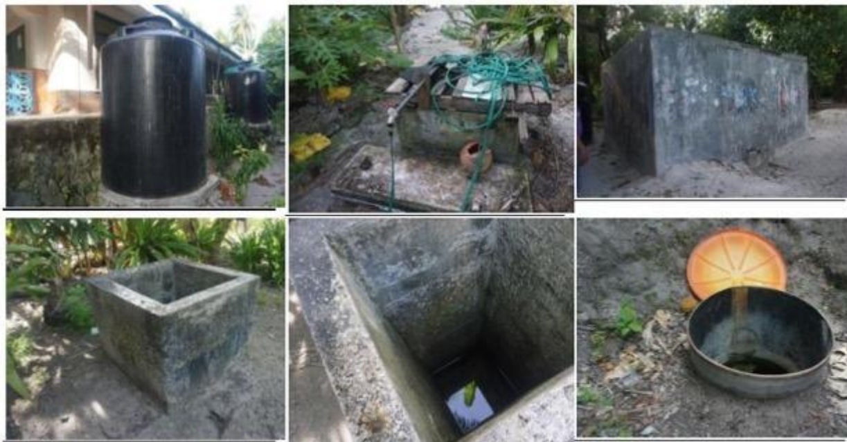
Figure 4. Sample of water tanks and wells from outer islands – Eauripik, Woleai atoll, Ifalik, and Feraulap atoll
