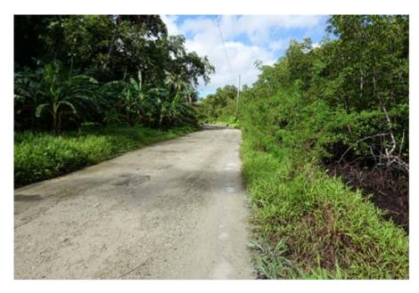
Figure 14: PACC road in Tafunsak completed to sub-base surface standard.
