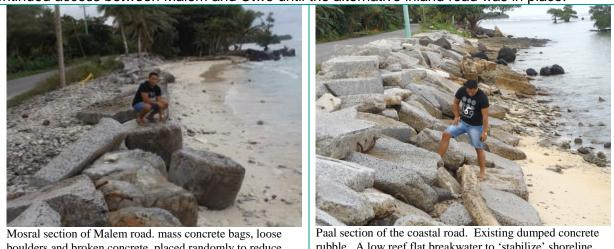
Mosral section of Malem road. mass concrete bags, loose boulders and broken concrete, placed randomly to reduce surge impact and prevent wave overtopping and erosion of road (photo credit: Simpson Abraham, 2015)
