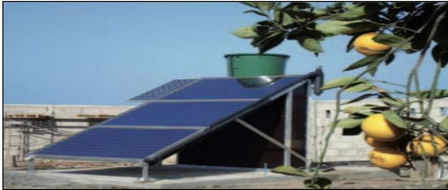
Figure 4: Membrane Distillation installed by SOLARSPRING GMBH
