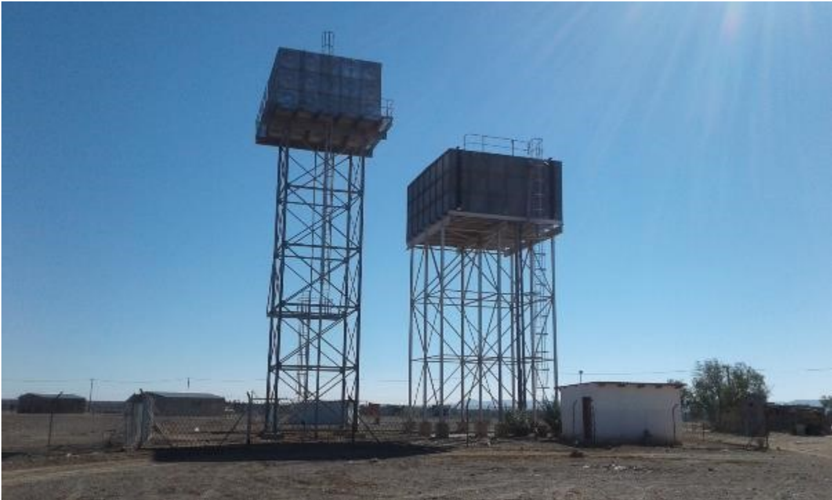
Figure 4: Water tank at Bethanie
