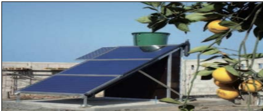
Figure 4: Membrane Distillation installed by SOLARSPRING GMBH
