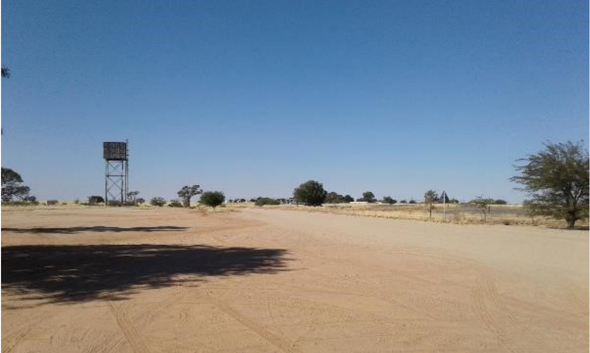
Figure 5: Water tank at Grünau
