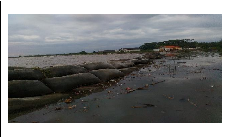
Coastal embankment with sediment/sand trap system
