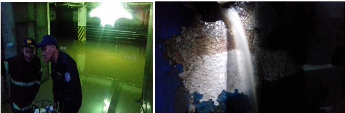
Basement of the 12 th apartment of Khilchin hothon – flood water and ground-water penetrating from the walls and floors leading to power cut restriction of 670 households Photo (UN-Habitat June 2017)
