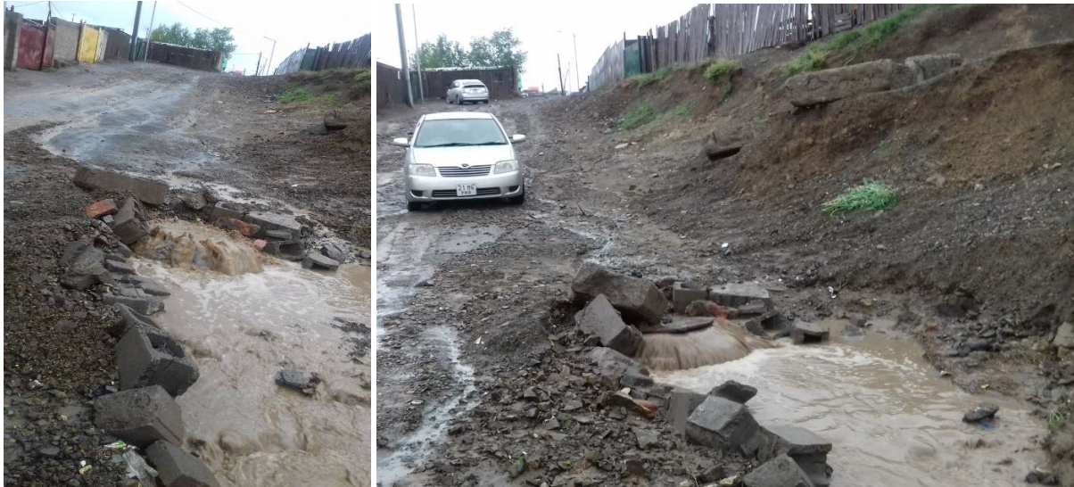
Flooding of main road sinkhole constructed by the Geodetic Water Facility Office of the Housing Authority Photo (UN-Habitat June 2017)
