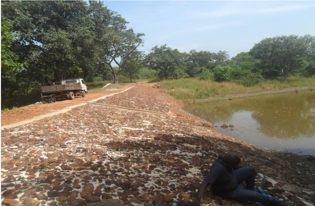
Partial view of micro dam (with a downstream water drainage channel) built in Bajocunda at the end of 2016 to control flood and used like a bridge
