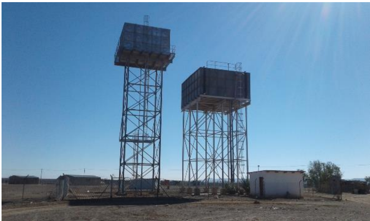
Figure 4: Water tank at Bethanie
