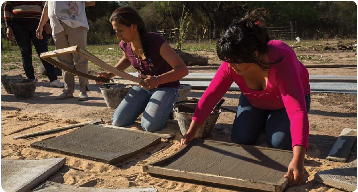
⌘ Beneficiaries of the project located in the province of Chaco, in the middle of construction of a cistern of 16,000 liters, destined to the capture of rainwater. Photo by Rodrigo Alonso
