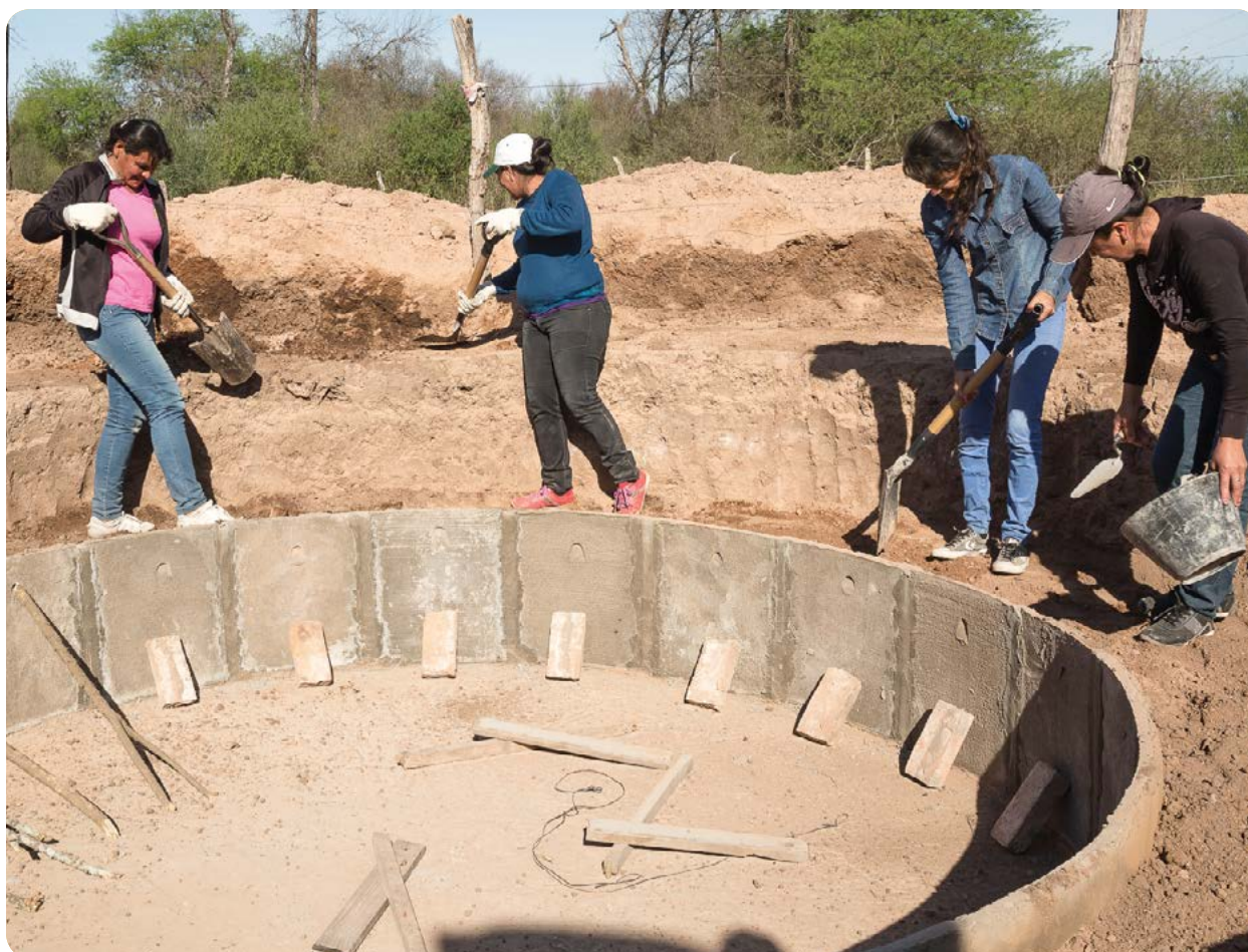
⌘ Beneficiaries of the project located in the province of Chaco, in the middle of construction of a cistern of 16,000 liters, destined to the capture of rainwater. Photo by Rodrigo Alonso, (UCAR)
