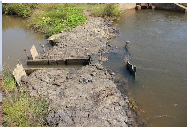
Figure 9. Insufficient and damaged water gate to protect rice fields from saltwater intrusion.
