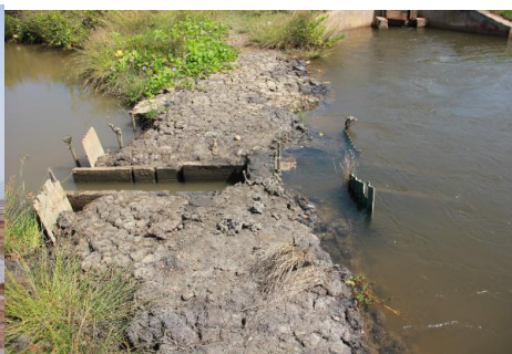
Figure 9. Insufficient and damaged water gate to protect rice fields from saltwater intrusion.
