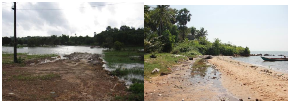
Figure 17. Beach erosion caused by sea-level rising and coastal storms.
