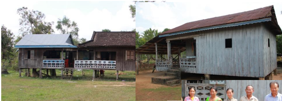
Figure 10: Re-construction of commune house after strong wind with limited resilience to impact.
