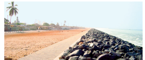
Seawall has been built in Rufisque along the coastline of Thiawlene in Senegal against coastal erosion. (Photo by CSE)
